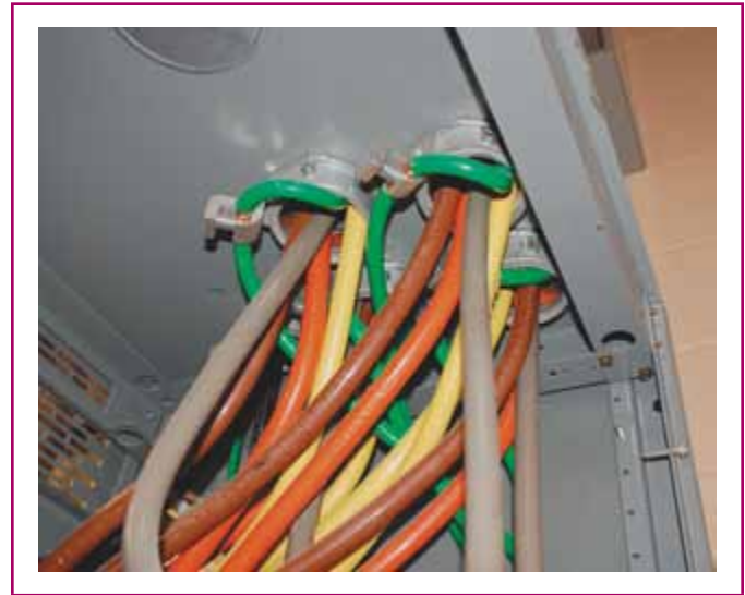
EXHIBIT 215.3 Different colors being used to identify each ungrounded line or phase conductor of a nominal voltage system.
