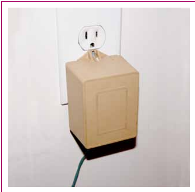
EXHIBIT 760.4 Duplex receptacle supplied by circuit dedicated to fire alarm equipment. (Courtesy of Merton Bunker)
