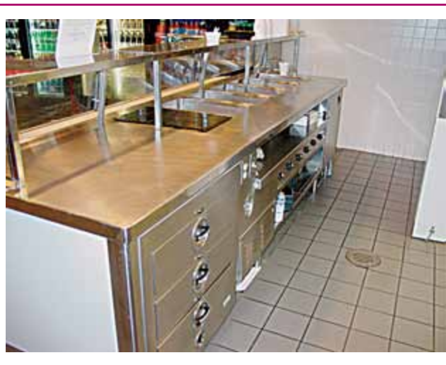
EXHIBIT 220.7 Electrically powered cooking/heating appliance with thermostatic control in a commercial kitchen. (Courtesy of the International Association of Electrical Inspectors)
