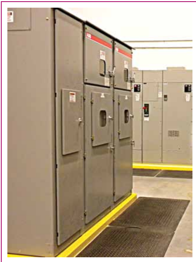
EXHIBIT 110.28 Medium voltage switchgear.
