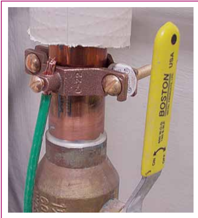
EXHIBIT 250.31 An application of a listed ground clamp.
