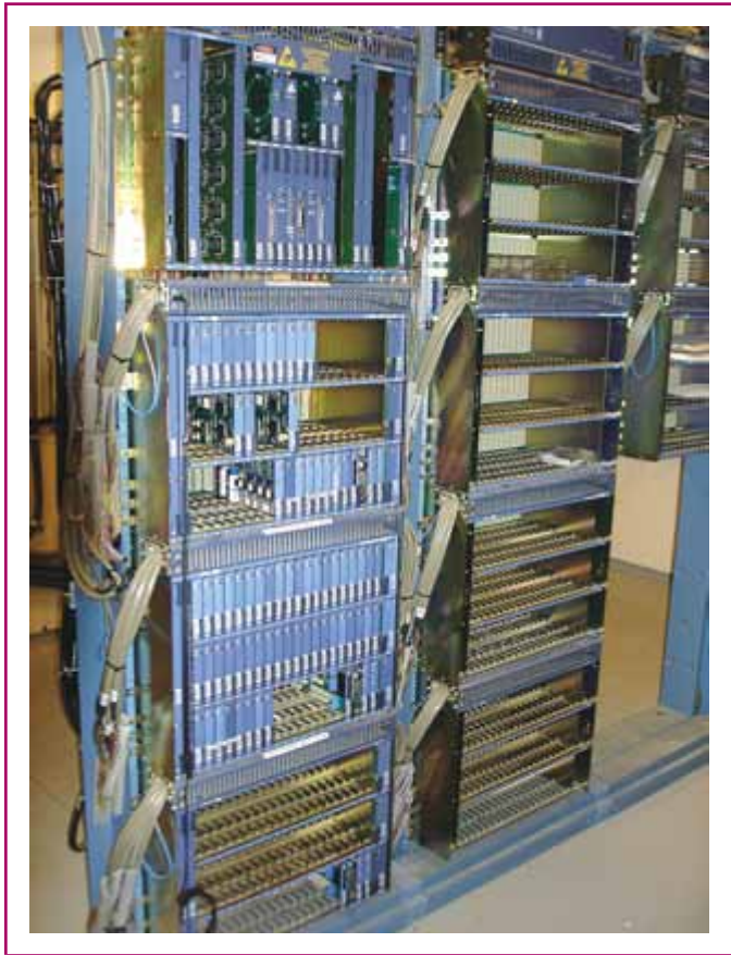
EXHIBIT 800.1 A private automatic branch exchange, which is one part of telecommunications equipment.
