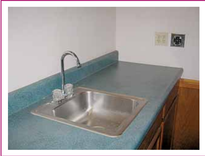
EXHIBIT 210.16 GFCI protection required for single-phase, 125-volt, and 250-volt, 15-ampere duplex receptacles installed within 6 feet of a sink if the receptacles are rated 50 amperes or less.
