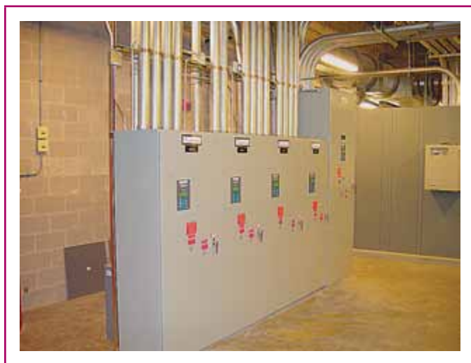
EXHIBIT 110.17 An equipment location that is free of storage to allow the equipment to be worked on safely. (Courtesy of the International Association of Electrical Inspectors)
