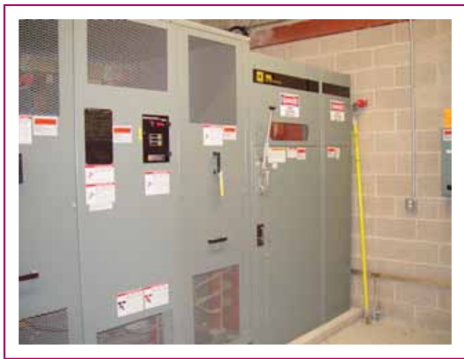
EXHIBIT 110.29 Enclosures of equipment operations at over 1000 volts required to have the warning label specified in 110.31(B)(1) . (Courtesy of the International Association of Electrical Inspectors)
