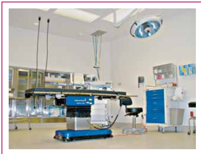
EXHIBIT 517.1 An operating room where patients are connected to line-operated electromedical devices while undergoing invasive procedures. (Courtesy of the International Association of Electrical Inspectors)
