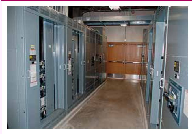
EXHIBIT 110.23 An installation of large equipment showing one of the required exits. (Courtesy of the International Association of Electrical Inspectors)
