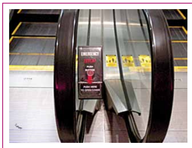
EXHIBIT 620.5 The emergency stop button installed at the escalator location is not considered to be the required disconnecting means.
