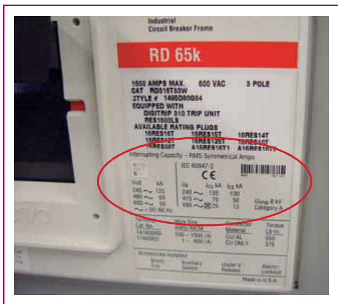
EXHIBIT 100.12 Interrupting ratings information on the label of a 1600-ampere frame circuit breaker.
