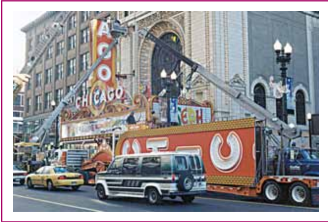
EXHIBIT 600.1 Example of a section sign where the subassemblies are field assembled to form a single sign. (Courtesy of Kieffer & Co. Inc.)
