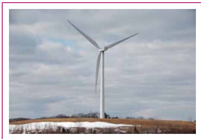
EXHIBIT 694.1 A wind electric system consisting of a single wind turbine.
