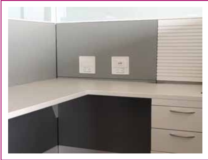
EXHIBIT 605.1 Example of a fixed-type office partition where the branch-circuit wiring is run inside the partition.
