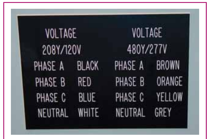
EXHIBIT 200.3 A label on a piece of equipment containing conductors of two nominal voltage systems that provides the required identification of the two systems.
