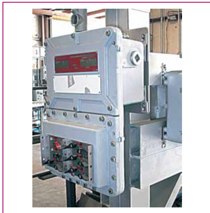
EXHIBIT 501.13 An explosionproof panelboard. (Courtesy of Appleton®, Emerson Electric Co.)
