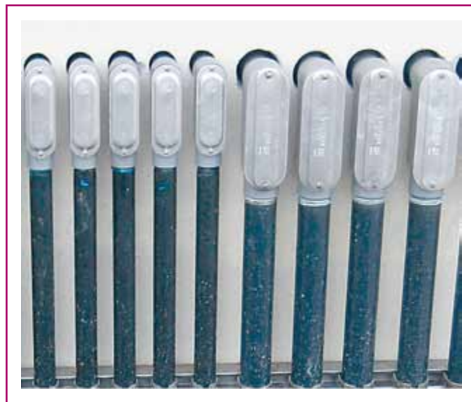
EXHIBIT 100.9 Typical conduit bodies. (Courtesy of the National Electrical Contractors Association)
