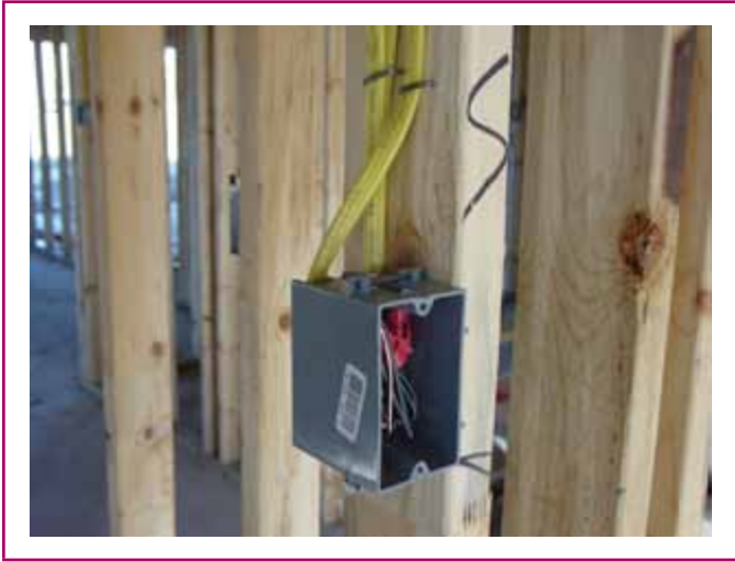
EXHIBIT 314.5 Installation of a single gang outlet with cables securely fastened within 8 inches of the box. (Courtesy of the International Association of Electrical Inspectors)
