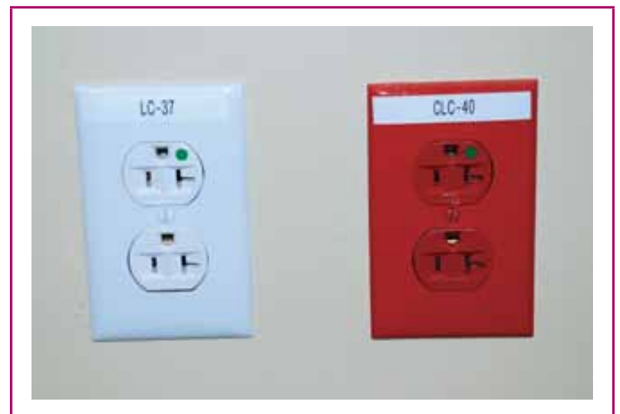
EXHIBIT 517.4 A receptacle from the normal system (left) and the critical branch (right). Note the label that indicates the panelboard and the circuit number. (Courtesy of the International Association of Electrical Inspectors)
