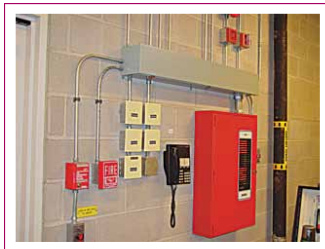
EXHIBIT 760.1 Typical fire alarm control unit. (Courtesy of the International Association of Electrical Inspectors)
