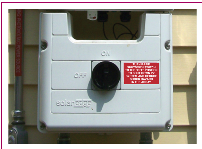
EXHIBIT 690.9 Rapid shutdown device.
