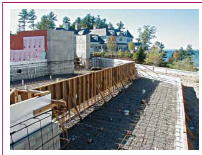
EXHIBIT 680.8 A poured-concrete pool with structural reinforcing steel that serves as the pool shell bonding grid.
