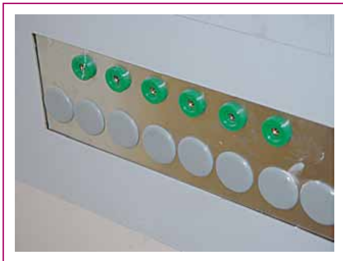
EXHIBIT 517.6 A patient equipment grounding point. (Courtesy of the International Association of Electrical Inspectors)
